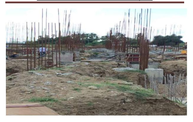
In Block D1: Excavation, Bar Bending & Shuttering for Pile cap work on Progress.
