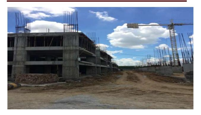
In Block C2: Excavation work, Shuttering for Short Column and for Pile cap Works on progress.
