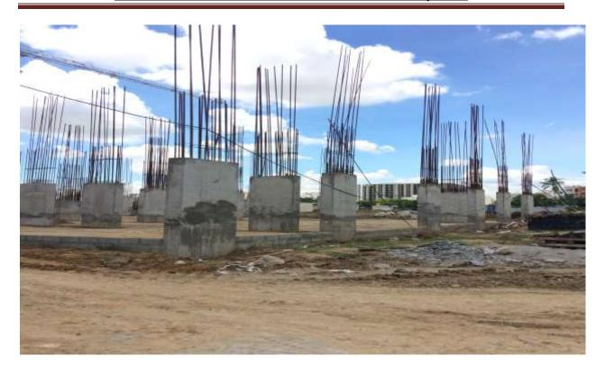
In Block C3: Excavation work for Pile Cap, Pile cap concrete Casting works on
