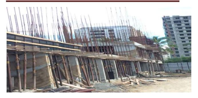
In Community Centre: Excavaion, Pile cap Concrete casting, pile chipping & Column Casing work on progress.
